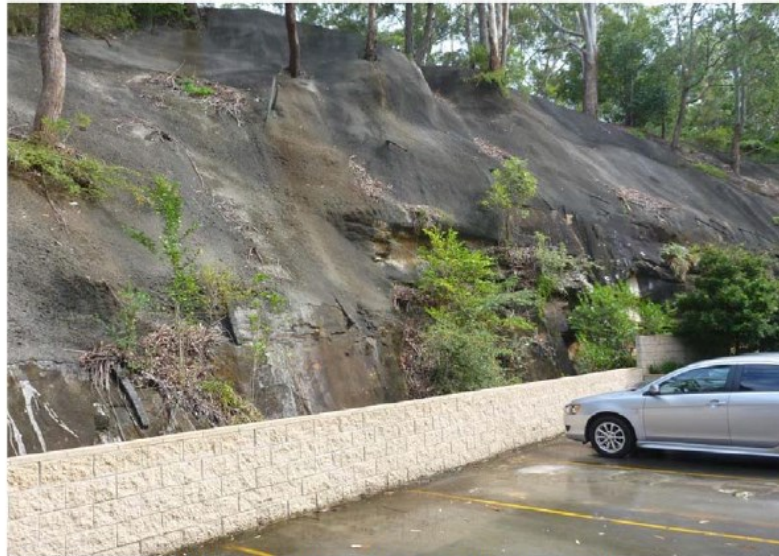
Photo 5 - Shotcrete slope in Area 2, at eastern boundary
