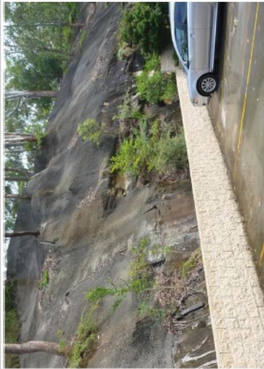
Photo 5 - Shotcrete slope in Area 2, at eastern boundary
